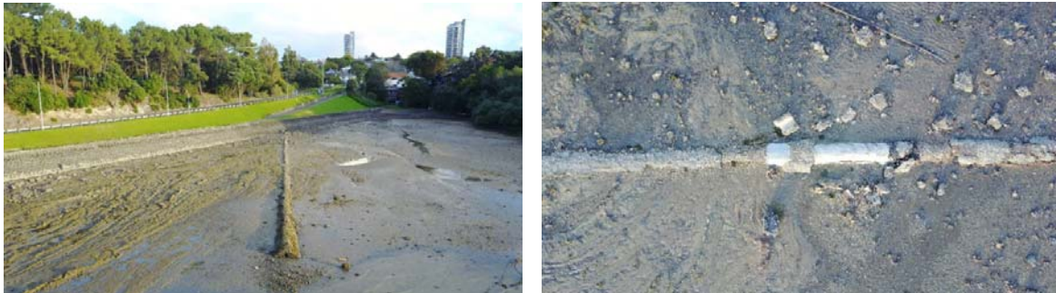
Photographs 1 and 2: The existing Masefield Beach failed outfall
